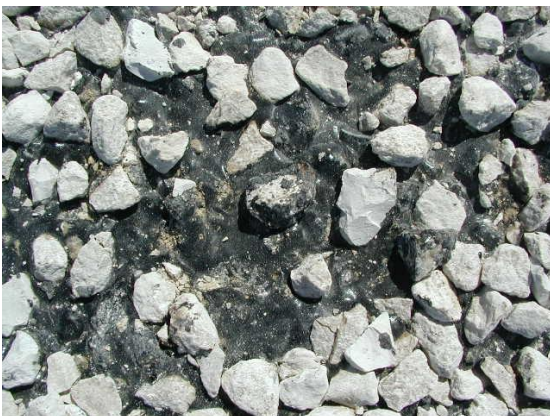
Insufficient aggregate.
