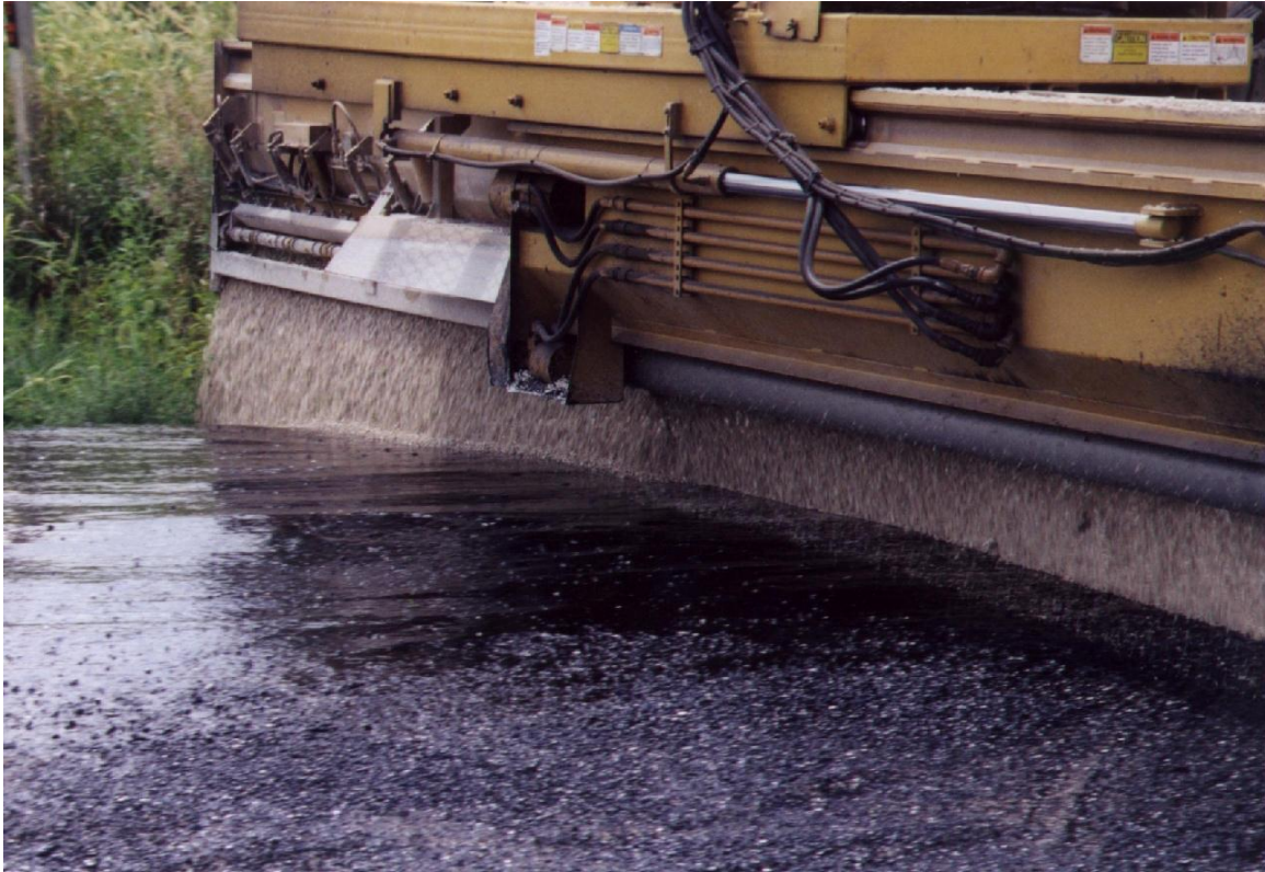
A uniform application of the aggregate.
