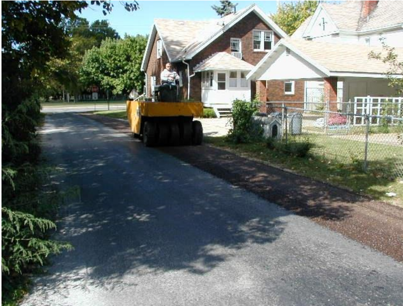
Roller ensuring proper embedment.
