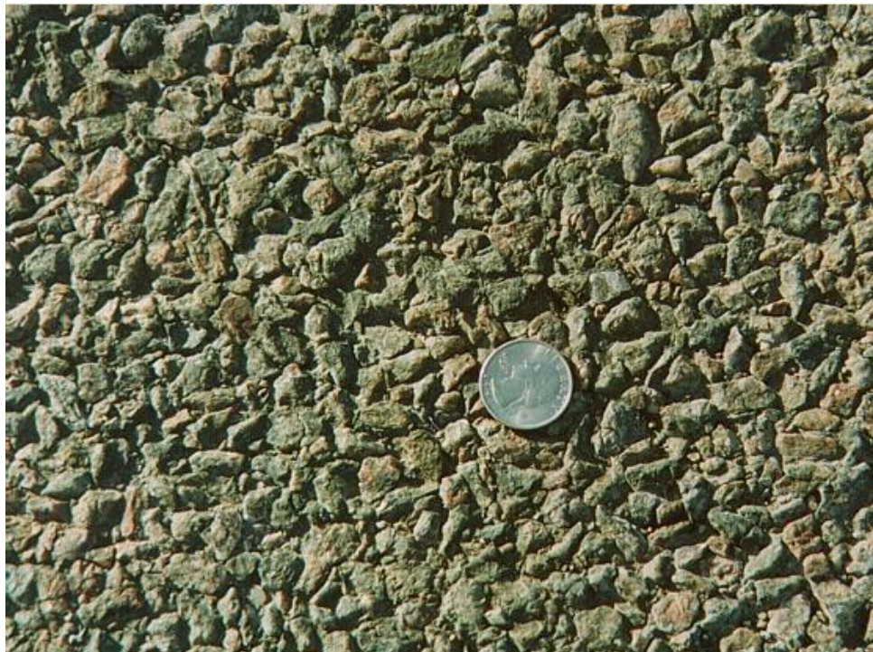
An open graded seal coat aggregate.
