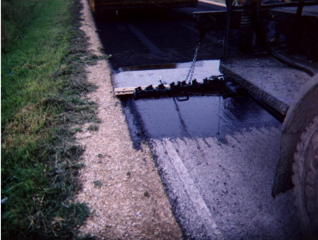
Slurry coat being applied to fill in alligator cracks.
