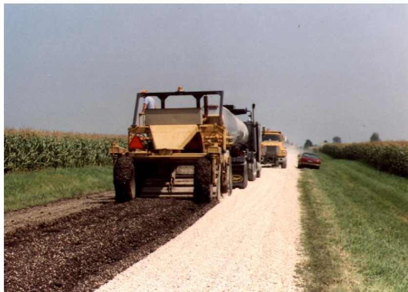
Tilling operation with new aggregate and bituminous material is added.
