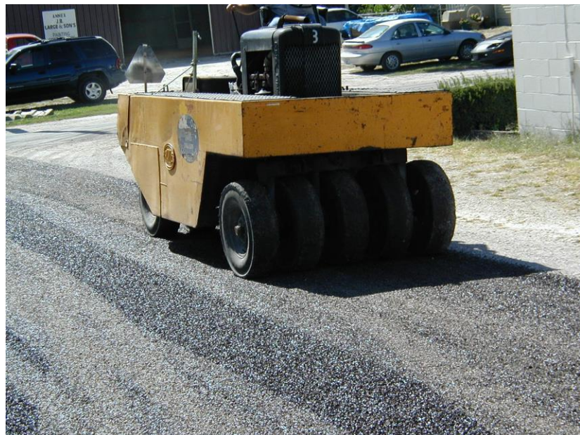
Tires should be free of asphalt to minimize chips from being dislodged.
