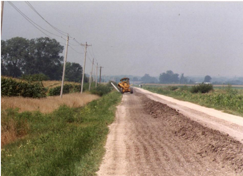
Scarifying and reshaping the road to correct defects, such as excessive crown.
