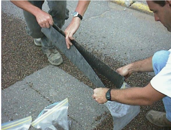
Here one foot strips are used to collect the aggregate.
