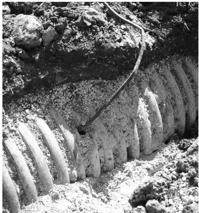
Culvert damaged by utility installation.
