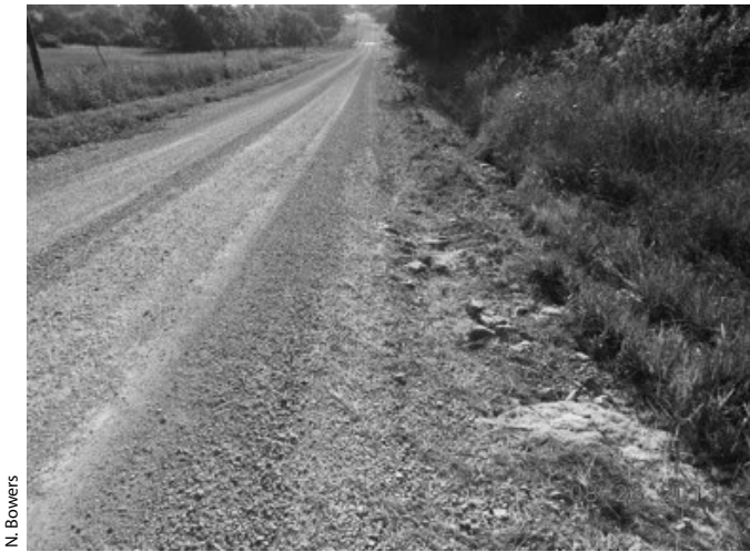
The “shoulder washing” evident at this site indicates the ditch needs to be larger to handle drainage.
