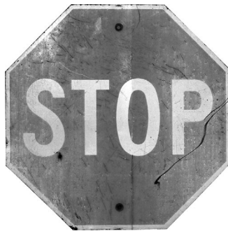
Improper signing or improper maintenance of signs is one of the easiest circumstances for a plaintiff to prove. The sign above is badly worn and should be replaced.
