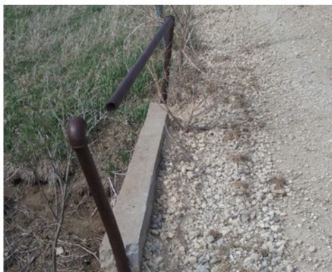
Figure 34: Ornamental concrete handrail may be removed to improve safety if the depth to the channel is less than 8 feet.
