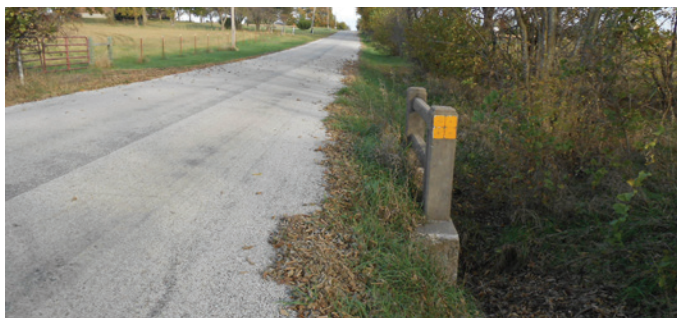
Figure 34: Ornamental concrete handrail may be removed to improve safety if the depth to the channel is less than 8 feet.
