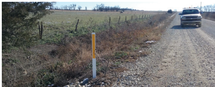
Figure 20: Flexible OM-2 for low volume roads with wide farm equipment
