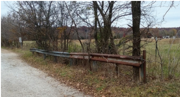
Figure 32: Old guardrail is probably more of a risk than trees and could be removed.
