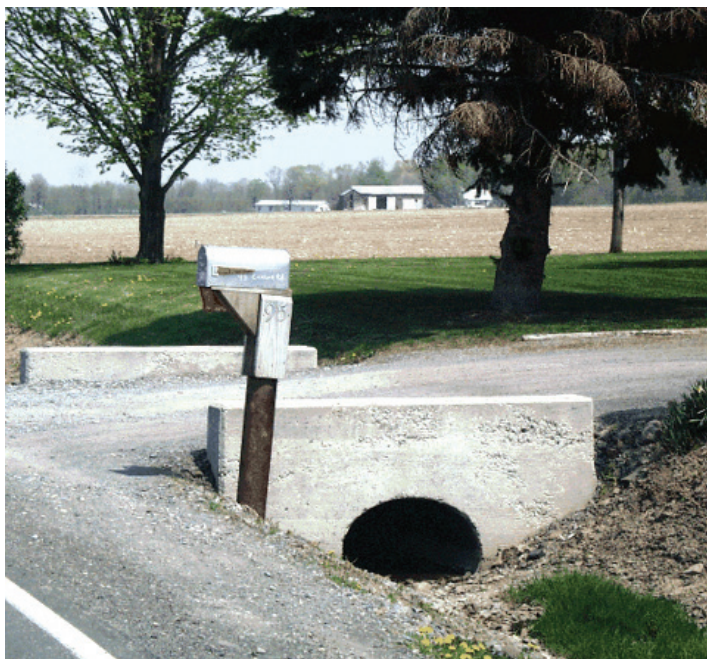
Figure 5: When an entrance culvert like this one needs to be replaced, the new culvert should have sloped ends.
