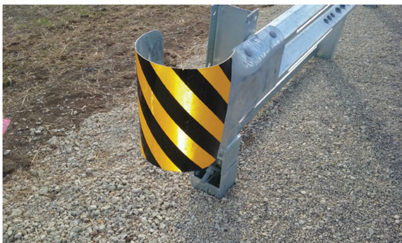
Figure 30: A buffer end shoe reduces chance of spearing
