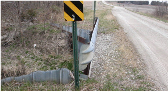
Figure 31: Guardrail is just ornamental and is a spearing risk which could be removed.
