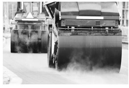
Paving crews are enthusiastic about Warm Mix Asphalt. Less smoke and less heat better than at the above Hot Mix project.
