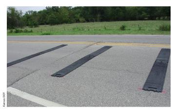
KDOT places the rumble strips in advance of the action warning sign at a work zone. The idea is that drivers will hit the strips and look up the see the sign.
