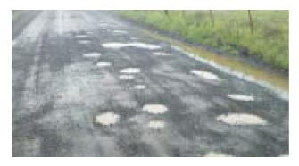
Fig 8. Potholes caused by inadequate cross slope at low spot in road.
