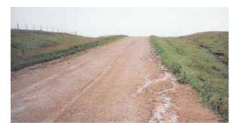
Fig 4. High shoulder causes erosion along edge of road.
