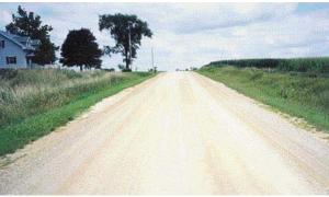
A well-maintained rock road has a four to six percent slope (crown) with a good crust and minimal loose material.
