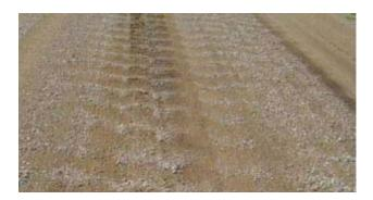
Fig 9. Washboards are common in dry weather.
