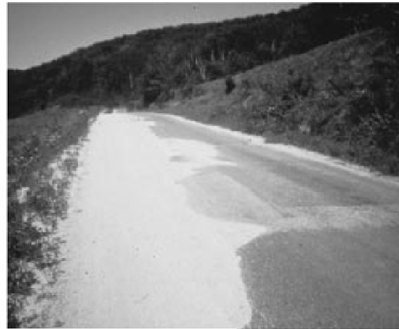
Figure 2. Sample PASER rating for asphalt pavement with rating of 5 (Walker et al. 2002).
