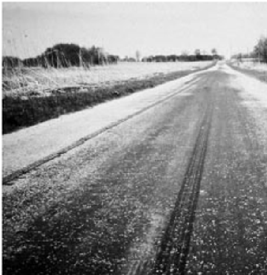
Figure 2. Sample PASER rating for asphalt pavement with rating of 5 (Walker et al. 2002).
