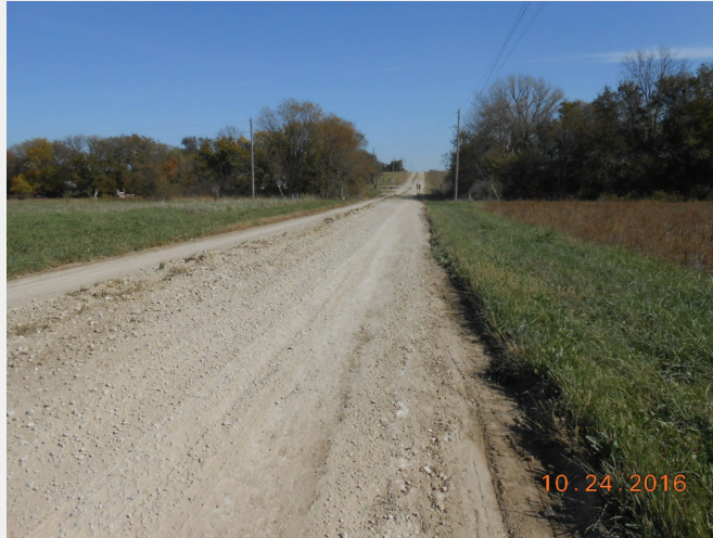
FIGURE 4: Worn blades result in high shoulders.
