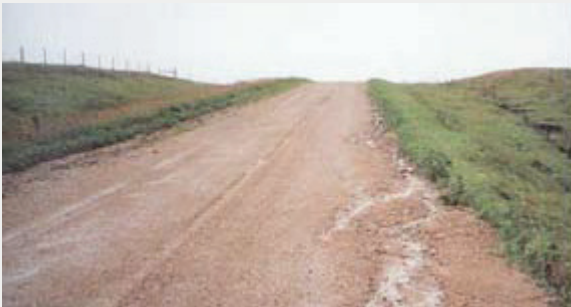
FIGURE 1: High shoulder accelerated by erosion along the edge of the road.
