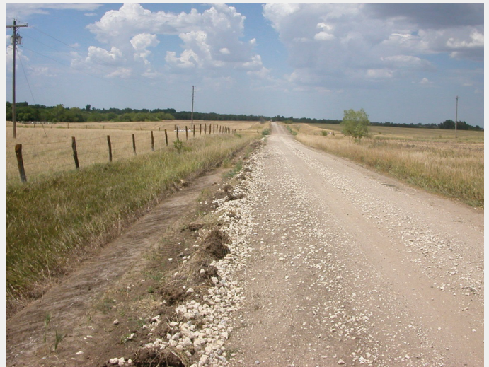
FIGURE 6: Pulling shoulders without mowing the grass or moving the windrow makes for a lousy job.
