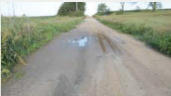
FIGURE 2: High shoulder results in mud hole at low area. Tall grass prevents grader from cutting off the shoulder.
