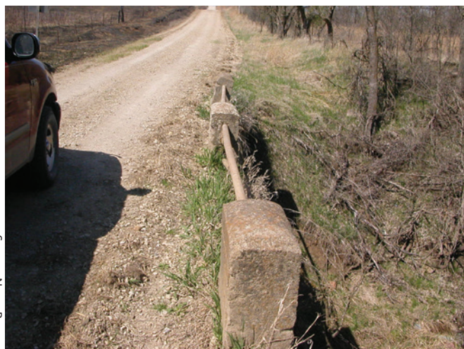
Figure 20. One example of many non-standard handrails constructed in Kansas pre 1950's.
