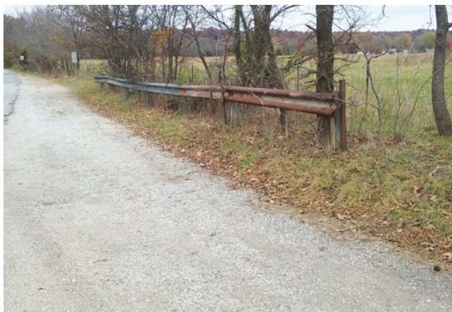
Figure 18. Guardrail is protecting the trees, not vehicles, and should be removed.
