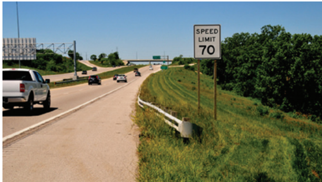
Figure 17. Guardrail that protects a gentle slope is more of a hazard than the slope.
