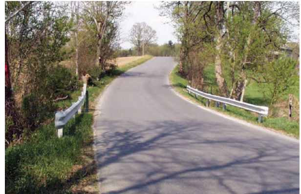
Figure 16. Old style guardrail with blunt ends and no spacers at posts.
