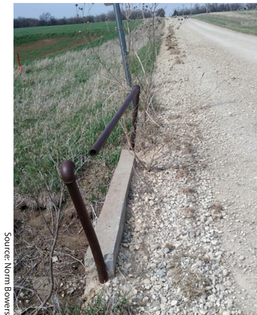
Figure 1. Pipe handrail is common in some areas and should be considered for removal.
