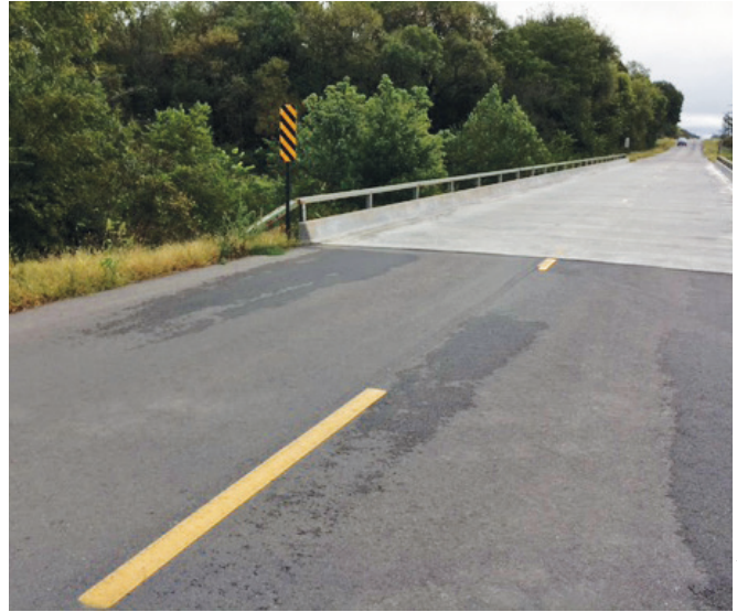
Figure 6. Structural steel used as handrail above a concrete curb.
