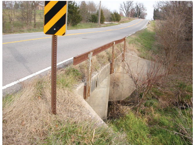
Figure 2. Steel handrail serves no purpose and could be removed.
