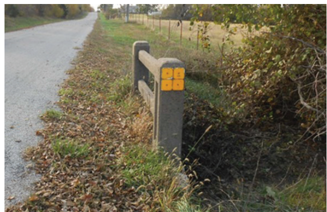
Figure 19. Standard post and beam concrete handrail could be removed to make a safer roadside.
