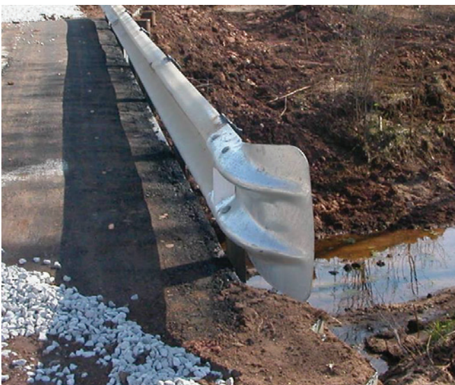
Figure 5. W-beam guardrail used for bridge handrail.
