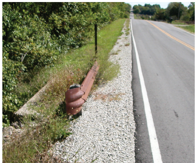
Figure 3. W-beam guardrail serves no purpose and should be considered for removal.
