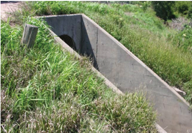
Figure 24. One of many variations of culvert openings.
