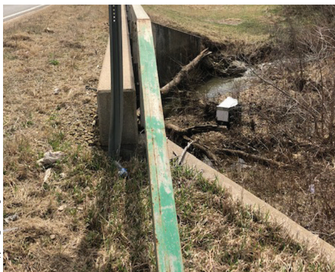
Figure 8. Bridge rail bent down to retard spearing.
