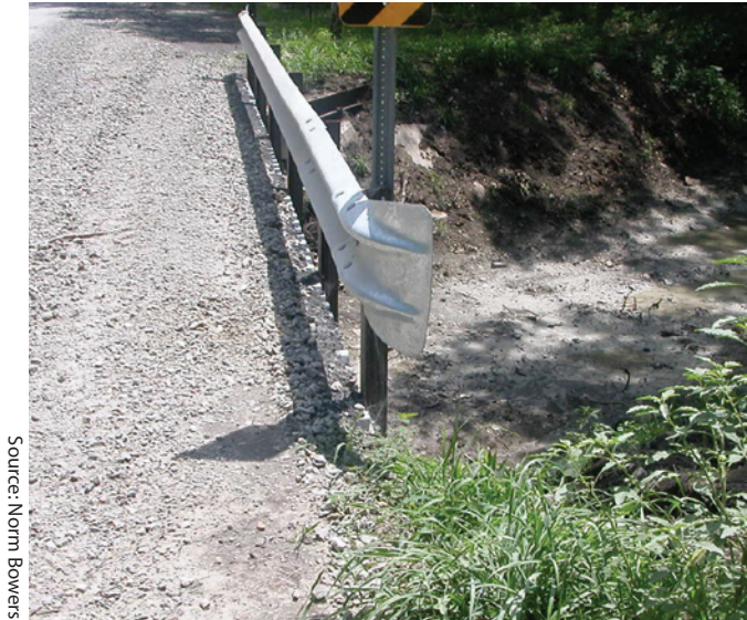
Figure 4. W-beam guardrail on a newer culvert that could be removed to enhance safety.
