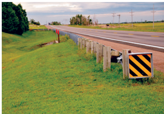
Figure 21. Guardrail protecting a culvert opening.
