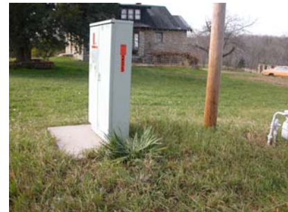
Figure 8. Large splice box in front yard.
