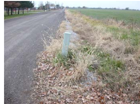
Figure 7. Splice box set over line at edge of shoulder.
