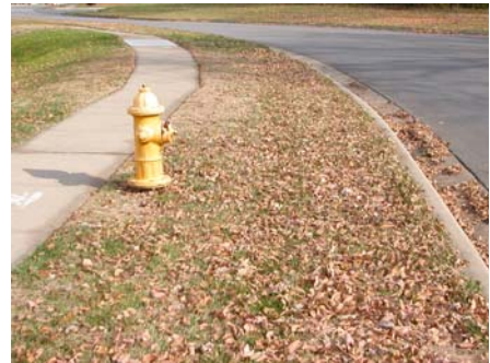
Figure 5. Fire hydrant set further back from curb.
