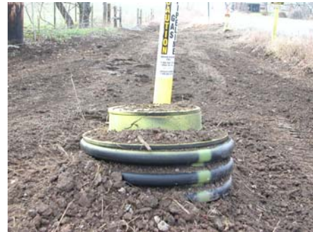
Figure 2. Water meter in clear zone improperly set too high.
