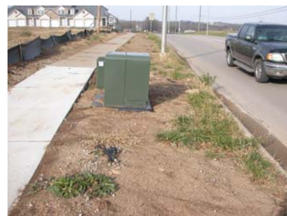
Figure 1. Power box set close to street due to lack of adequate easement behind the sidewalk.
