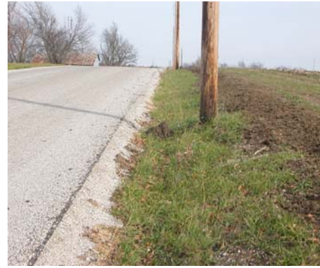
Figure 6. Power poles set close to road to avoid buried lines near the r/w line.
