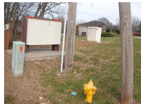
Figure 9. Large splice box and cabinets in front yard.
