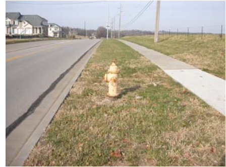
Figure 4. Fire hydrant set too close to curb.
