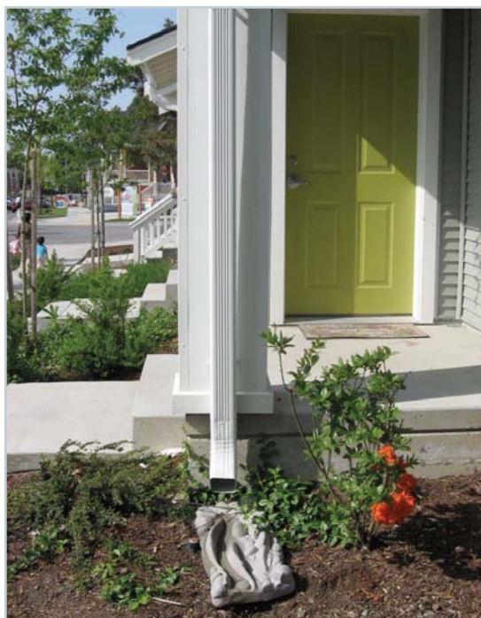
Figure 13: A disconnected downspout in Seattle, Washington.
