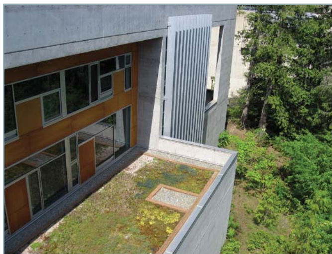
Figure 1: A green roof at Evergreen College was built to offset the addition of new impervious surfaces from new parking spaces.
