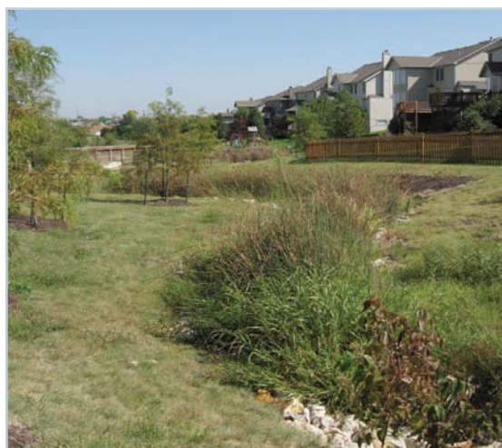
Figure 1: A constructed 1 st order intermittent stream in a neighborhood development slows and infiltrates stormwater runoff, while adding aesthetic value for residents. Plant selection and landscape transition plantings were carefully considered for acceptance.
