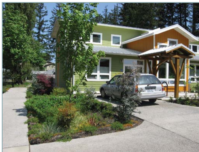
Figure 2: A medical center in Olympia, Washington, manages runoff from the roof and other impervious areas through small swales and permeable sidewalks.
