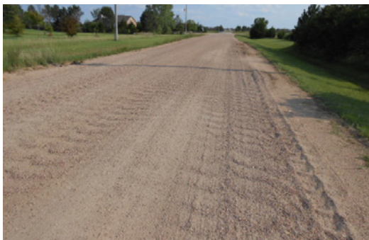
Figure 9-3. Washboards are caused by lack of cohesive binder and excess loose material on the road surface. (Source: Norm Bowers)
