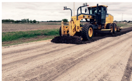
Figure 9-4. Washboard area being scarified with bullet blades to the bottom of the washboards. (Source: Pawnee County)
