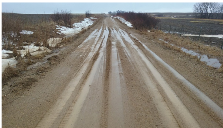
Figure 9-2. Rutting and mudholes caused by poor drainage including lack of crown, false shoulders, and windrow without weep holes. (Source: Norm Bowers)
