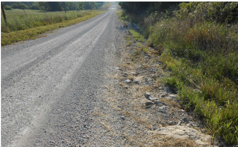
Figure 6-3. Washing of shoulder indicates inadequate ditch capacity. (Source: Norm Bowers)
