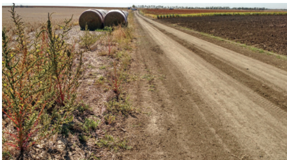
Figure 4-1. Hay bales in right-of-way obstruct wide farm equipment and can be a safety issue to errant vehicles. (Source: Marion County)
