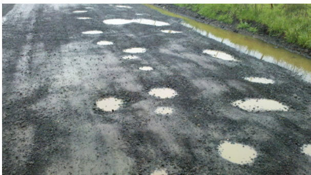
Figure 9-1. Inadequate crown is the major cause of potholed areas in a gravel road. (Source: Norm Bowers)
