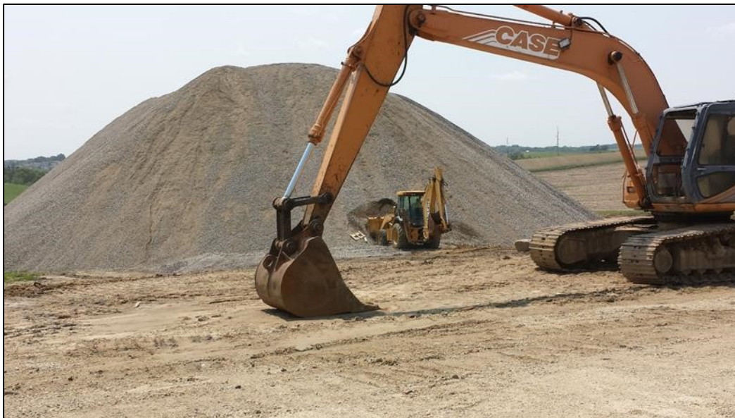
Figure 18. Recycled concrete aggregate (including fines) is obtained from a stockpile.
