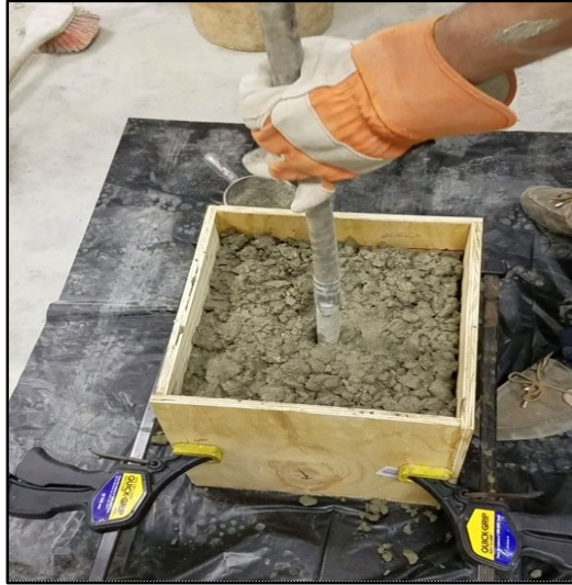
Figure 24. The concrete is vibrated for 3 seconds in and 3 seconds out.
