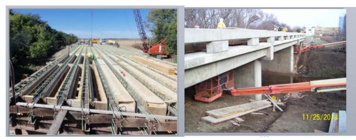
At left, placement of formwork and supplemental reinforcing around existing steel beams in preparation for concrete placement. At right, Removal of formwork after completion of concrete placement.
