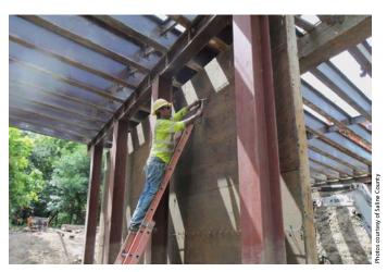
Construction of formwork for subsequent encasement of the open H-pile bents with concrete.
